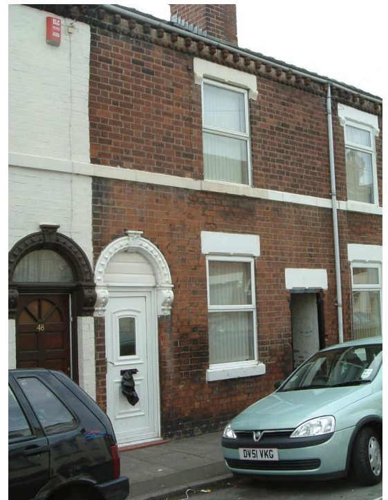
No. 46 Seaford Street, Shelton, Hanley – this is the only one of the many houses mentioned in Stoke which still exists!
